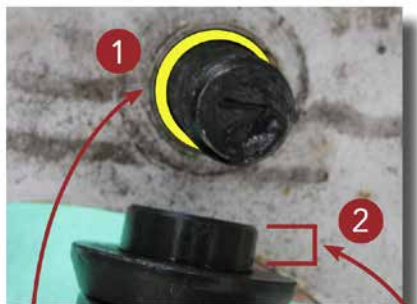
1) YELLOW HIGHLIGHT shows void between stud and stud hole. 2) Skirted Nut fills void between stud and hole.
