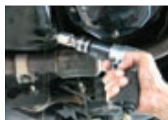
DRILLING DRAIN HOLE
